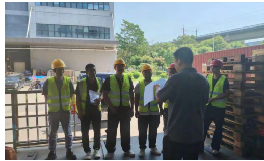
Contractor Pre-entry Safety Training On-site Photo
